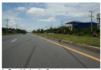
Figure 3-14: Yaw Marks Analysis Considering its Geometry
