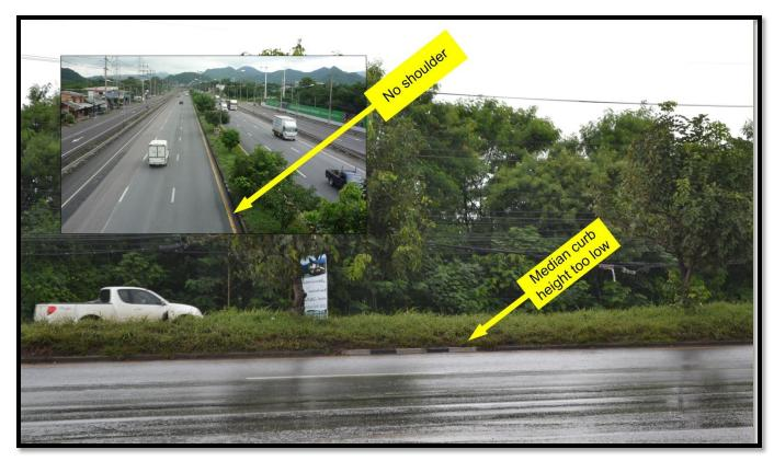
Figure 21 Low Height Median Curb and No Shoulder between Right lane and Median
