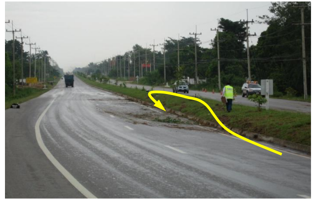
Upstream- Right Turn into the Curve
