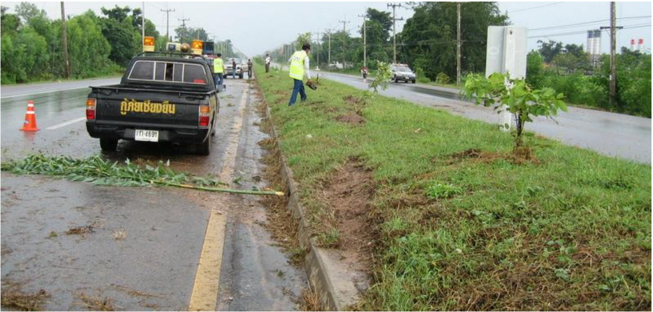
Figure 3-7: Evidence on the road
