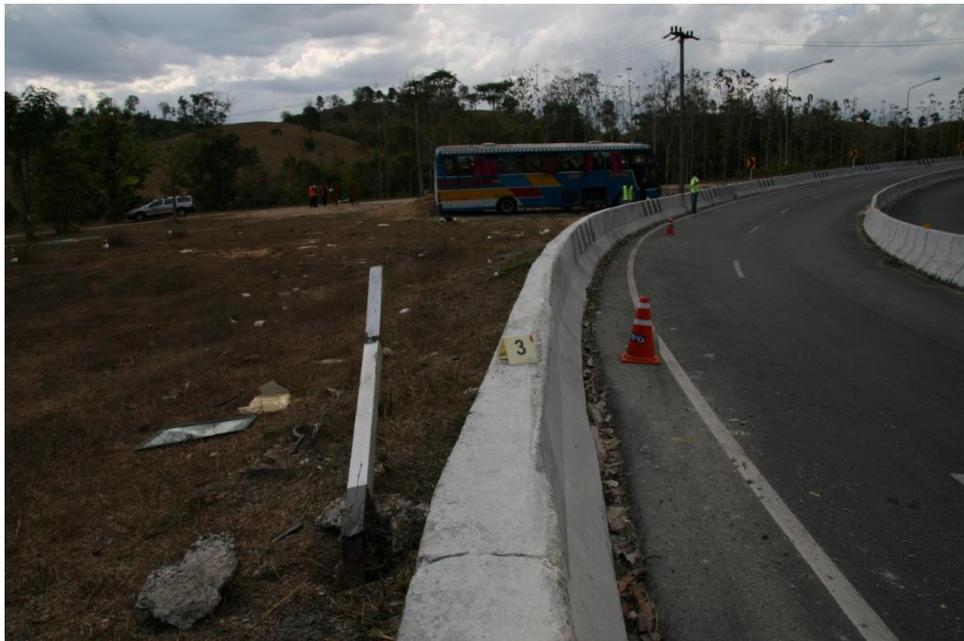
**Figure 3-25: The damages of Chevron Sign and Electric Post**
