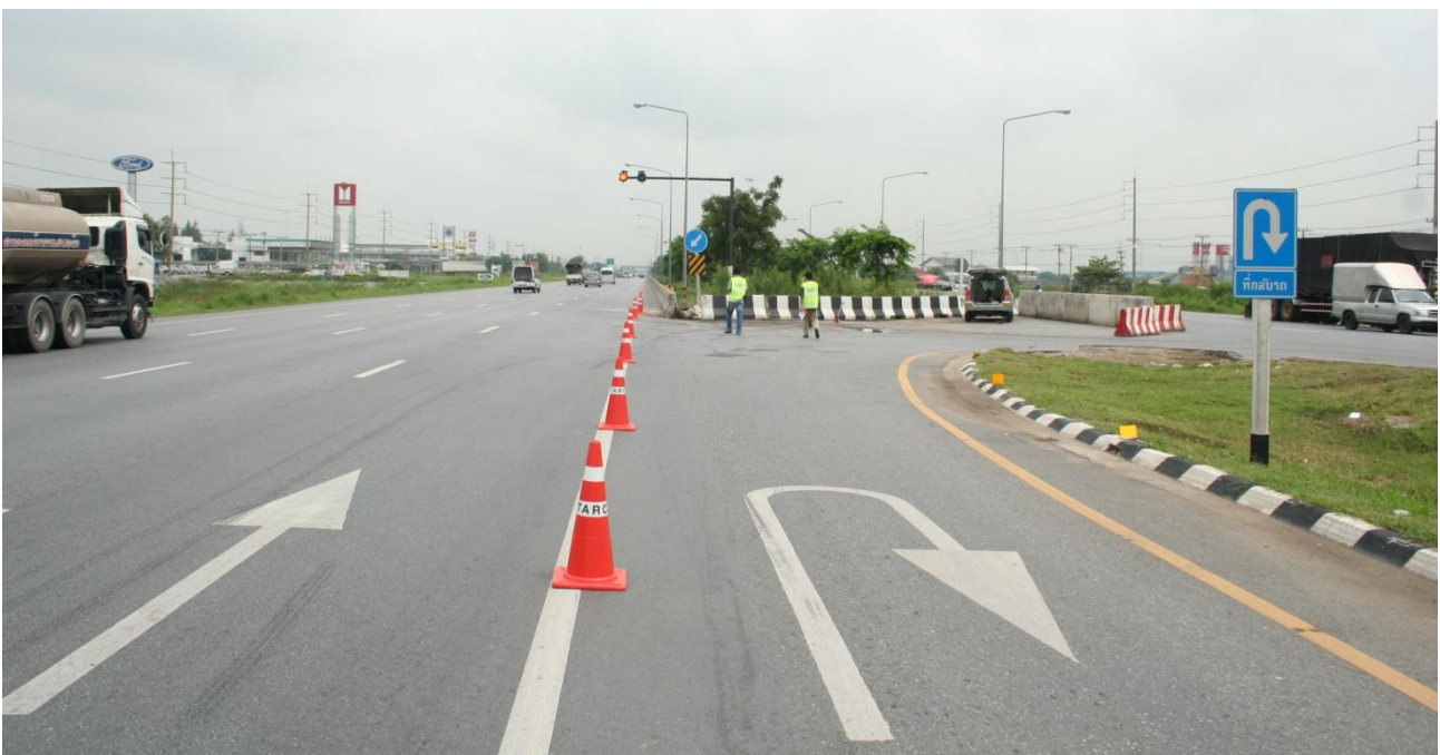
Figure 3-8: Median Opening U-Turn
