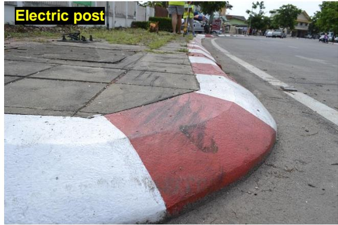
Figure 31 Tire marks of van on the curb
