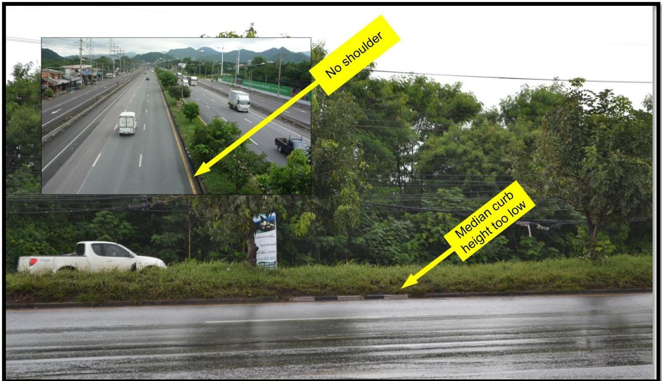
**Figure 21 Low Height Median Curb and No Shoulder between Right lane and Median**
